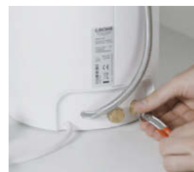
Connect boiler to safety group and tap. Afterwards open the angle valves before connecting power supply.
